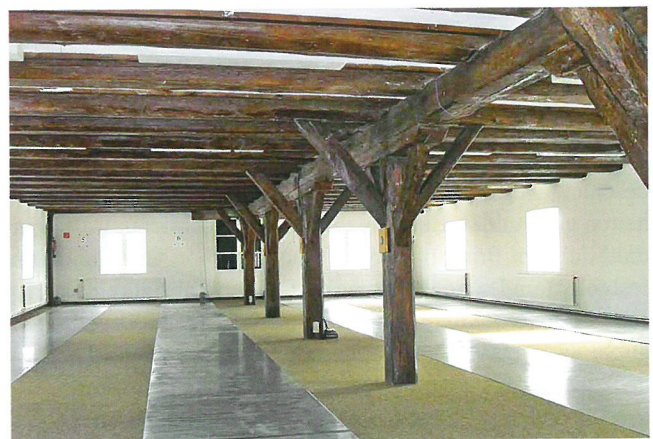
Abb. 5: Bremen, Vegesack, Thiele-Speicher um 1800, innen
